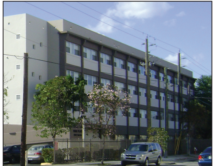
Park Place offers barrier-free rentals in Hialeah. More than half of the residents have a disability.
